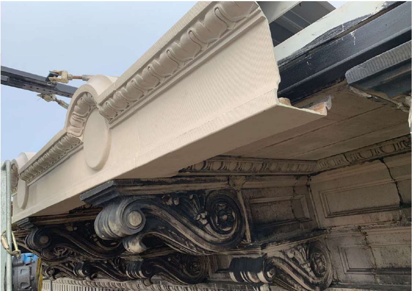
Figure 19. A new, lightweight fiber reinforced polymer is attached to a new metal armature to replicate damaged and missing elements of a terra cotta cornice. Photo: Quinn Evans.
