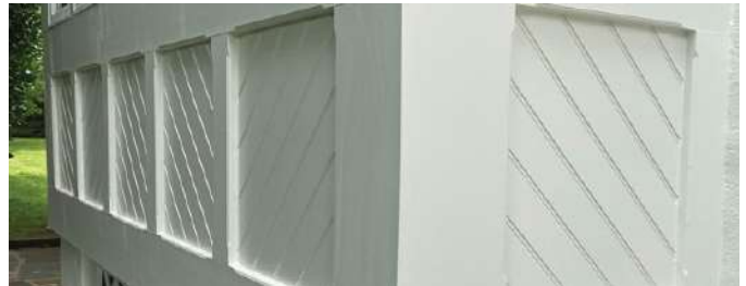
Figure 24. Cellular PVC when painted can be used to replace deteriorated wood features. This beadboard set in a wood frame was not historically designed to shed water effectively and had deteriorated. Cellular PVC was able to match the appearance of the wood details, while its properties were well matched to the shady location, painted finish, and limited size and configuration within the overall assembly; thus, it should provide a long-lasting solution for this application. Photo: Jennifer Balson Alvarez, NPS.
