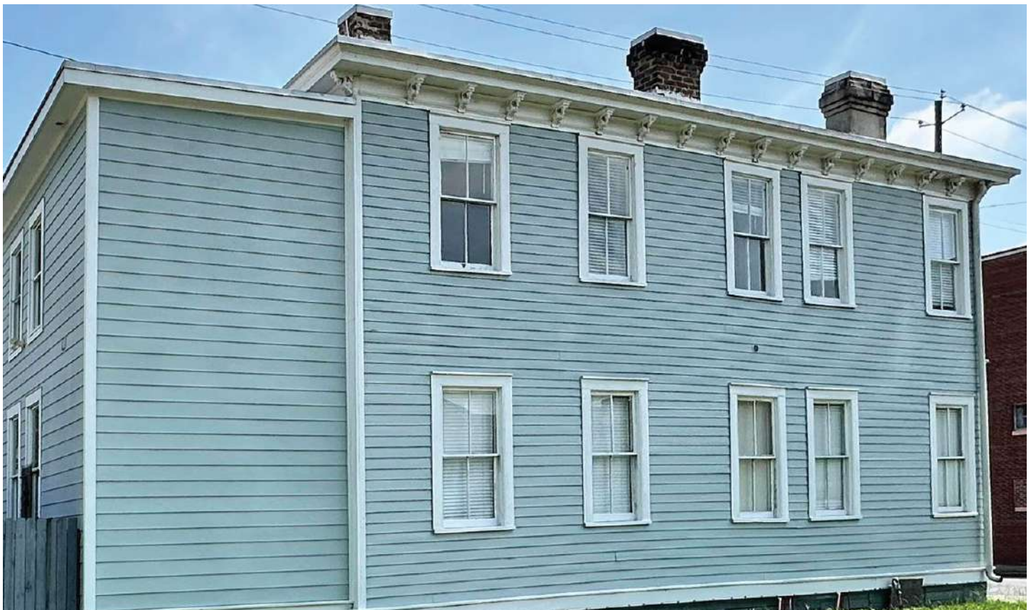
Figure 7. A new addition replaced non-historic construction on the rear elevation of this building. Fiber cement gives the addition a compatible appearance without replicating the exposure for thickness of the historic siding. Photo: Ward Architecture + Preservation.
